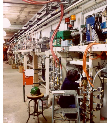
Figure 5: The trunkline during construction.
