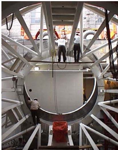
Figure 6: Installation of a 90 ton gantry.
