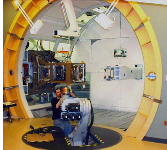
Figure 7: The Patient Positioning robot and DDS exposed during the final stages of construction. This is the view of a gantry from the Treatment Room.
